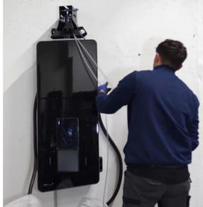
Figure 9: Lifting up the HYC50
